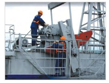
assembling and dismantling, commissioning and start-up works of sucker-rod pump drives;
